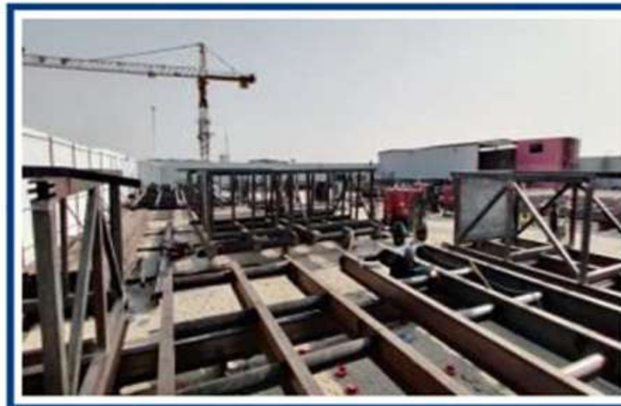
Machining, Fabrication & Erection
