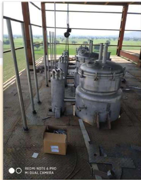
Milk Evaporator Plant
