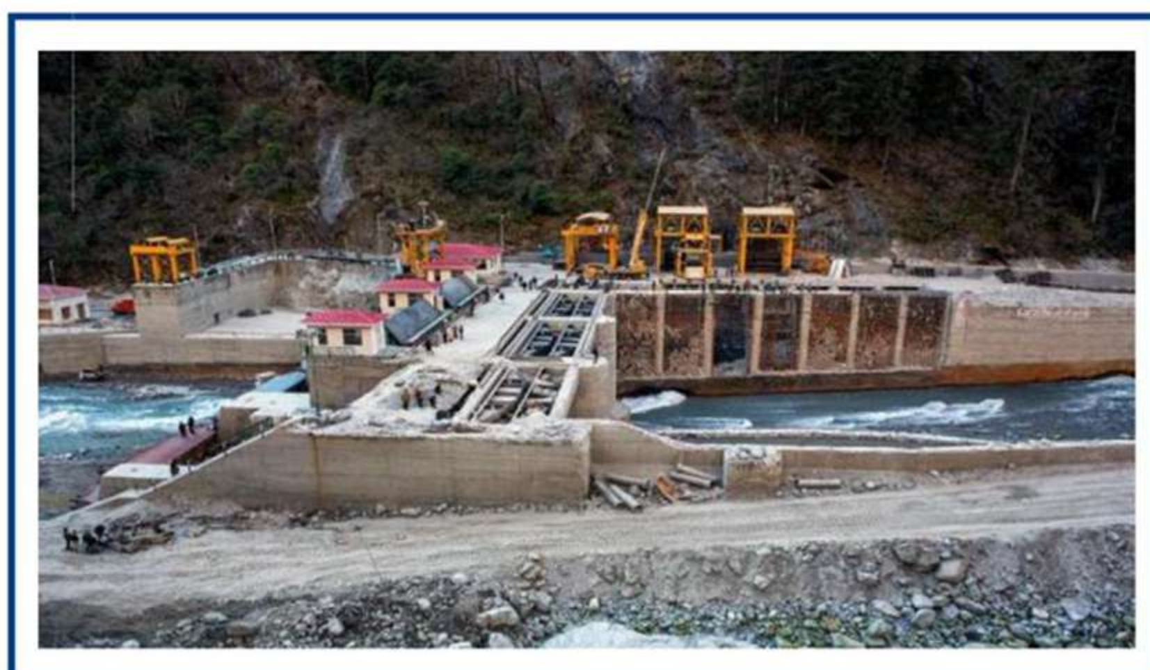
Vishnuprayad Hydroelectric Project
