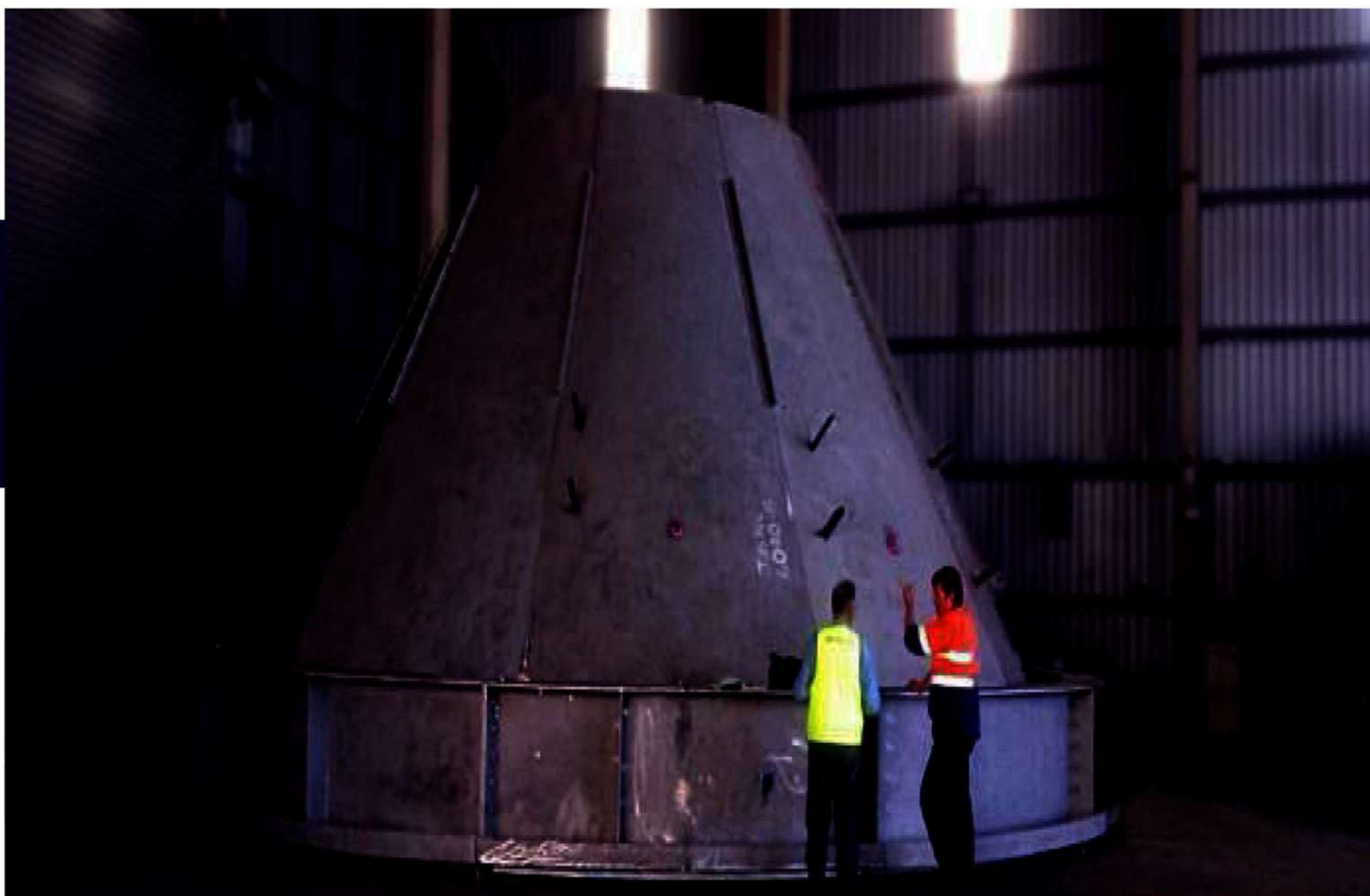
Fabrication at JSW Dolvi plant
